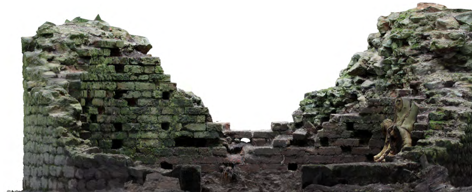
External West Facing Elevation of Garden Structure
