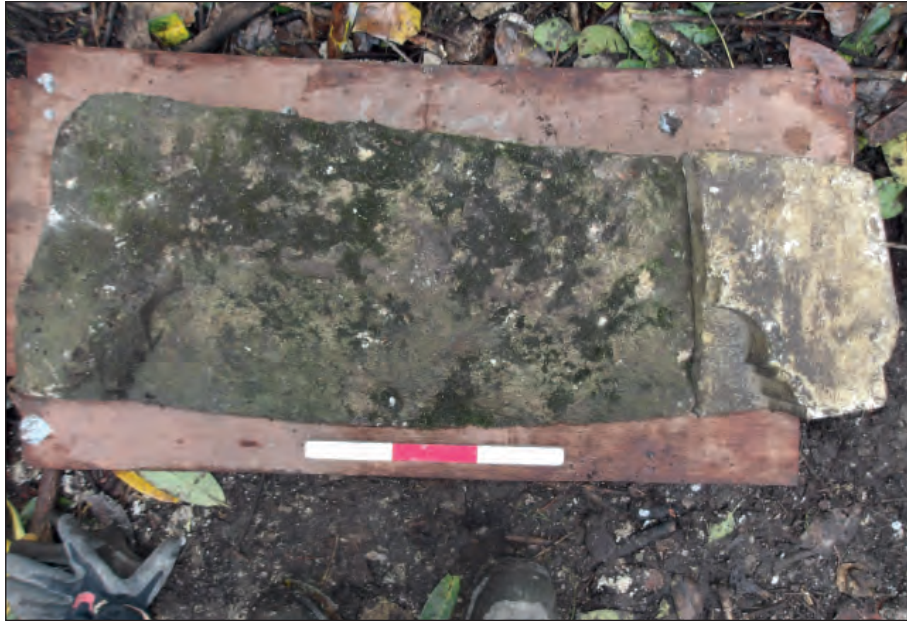
Figure 17: Stones 4 and 7: windowsill and reveal. 0.5 m scale
