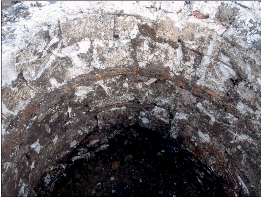
Plate 5: Detail of well 207, showing tile lacing courses
