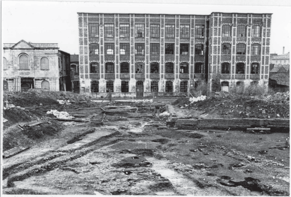
Plate 1. General view of the excavations, looking North towards Home Mills.
