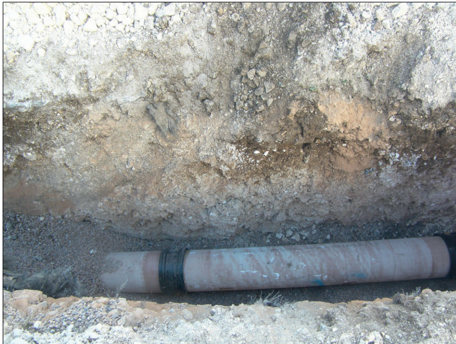
Plate 1: South-west facing section of the main Larkhill WWTW compound. Scale is 1 m
