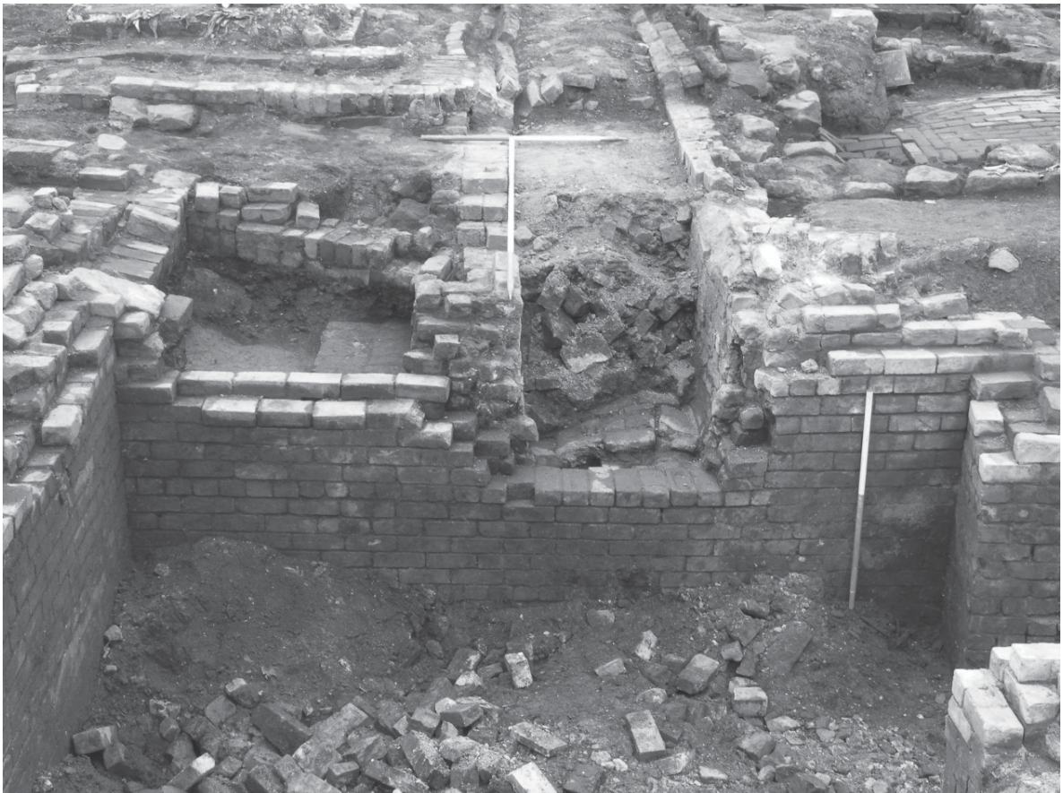
Plate 2: Building C, flues 7021 and 7032 beneath the furnace structure
