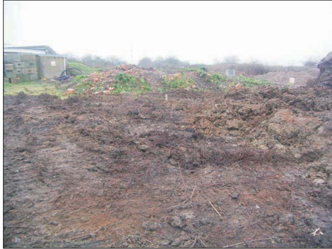
Plate 7: DAT Battery topsoil strip area B, view from east
