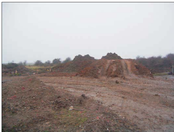
Plate 5: DAT Battery topsoil strip area A, view from south
