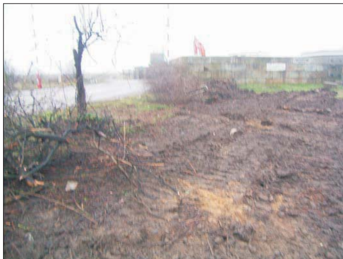
Plate 6: DAT Battery topsoil strip area B, view from east
