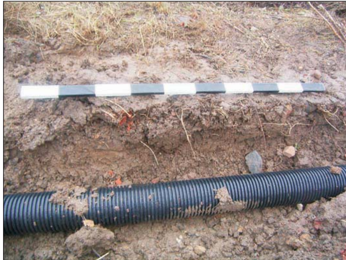
Plate 4: DAT Battery service trench, view from south
