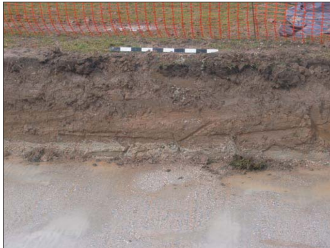
Plate 8: ETC Battery footings trench, view from south-east
