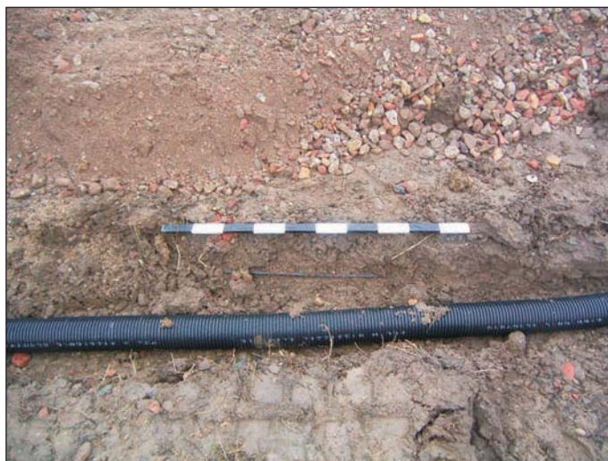
Plate 2: DAT Battery service trench, view from north
