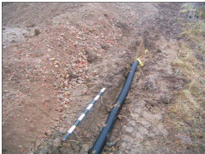
Plate 3: DAT Battery service trench, view from north-east
