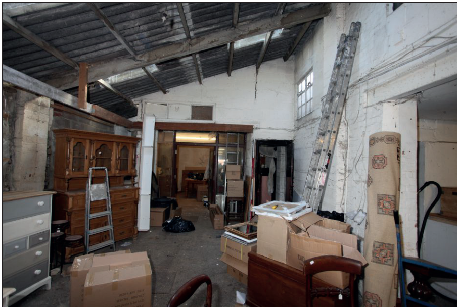
Plate 4: View of the central workshop of the lean-to, facing east
