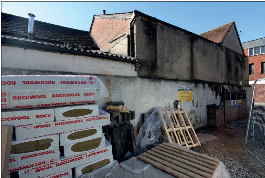
Plate 2: South-west facing view of the north, exterior elevation of the lean-to structure and 13 Brown Street
