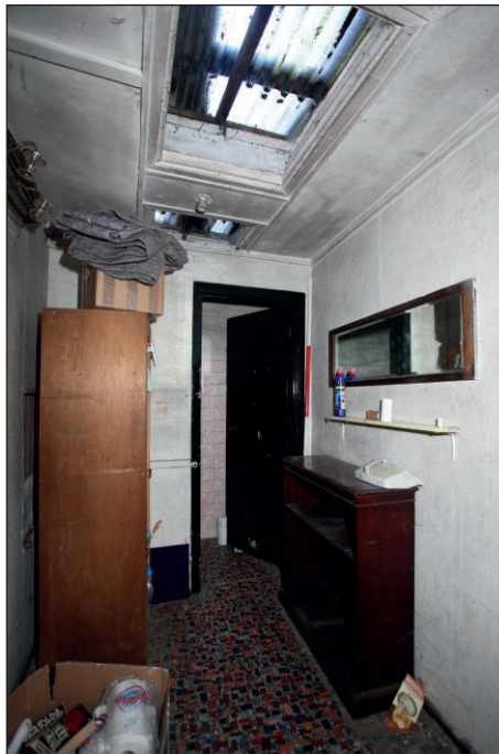
Plate 10: East-facing view showing the lean-to extension and the outer wall of the flat-roofed structure
